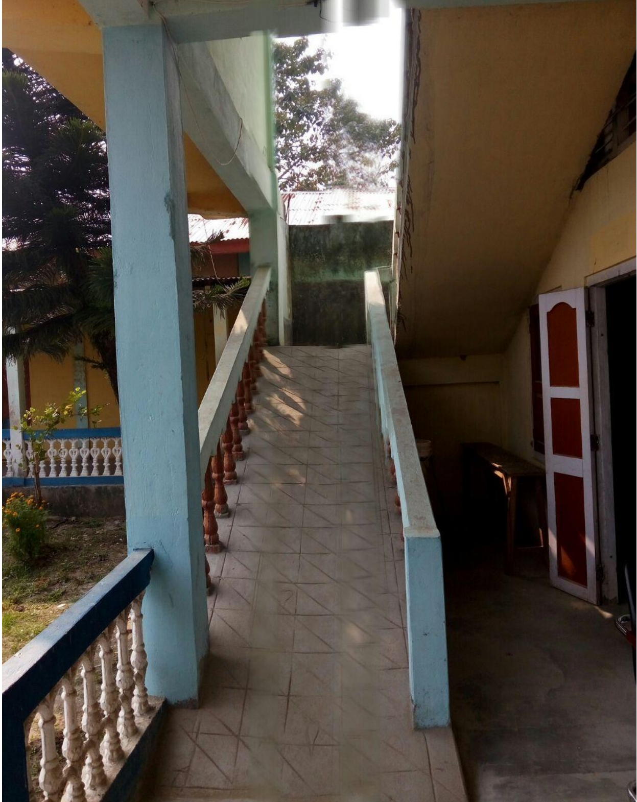
Staircase for Differently Abled Student in front of College Library
