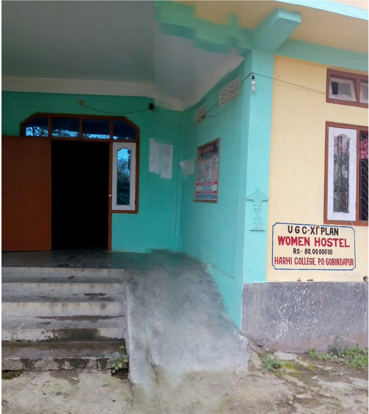
Staircase for Differently Abled Student in front of Girls' Hostel
