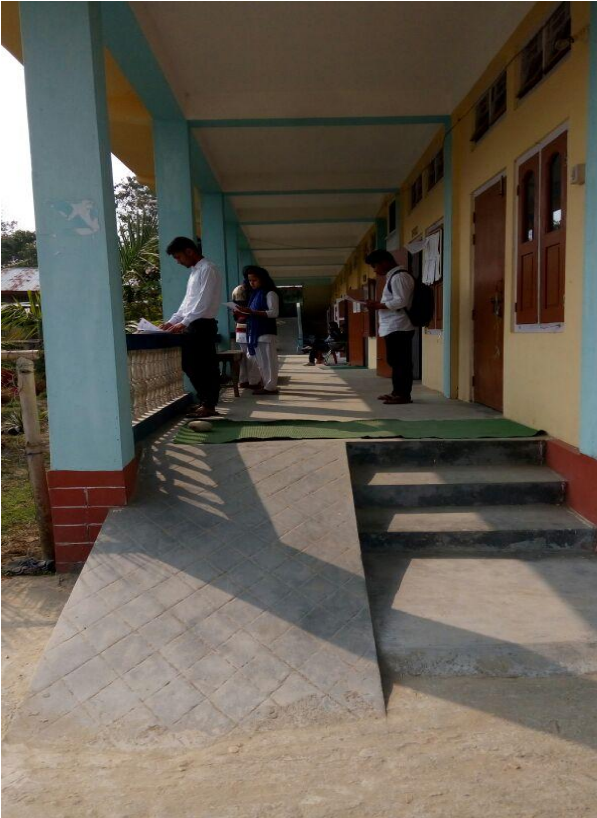
Staircase for Differently Abled Student at Administrative Building
