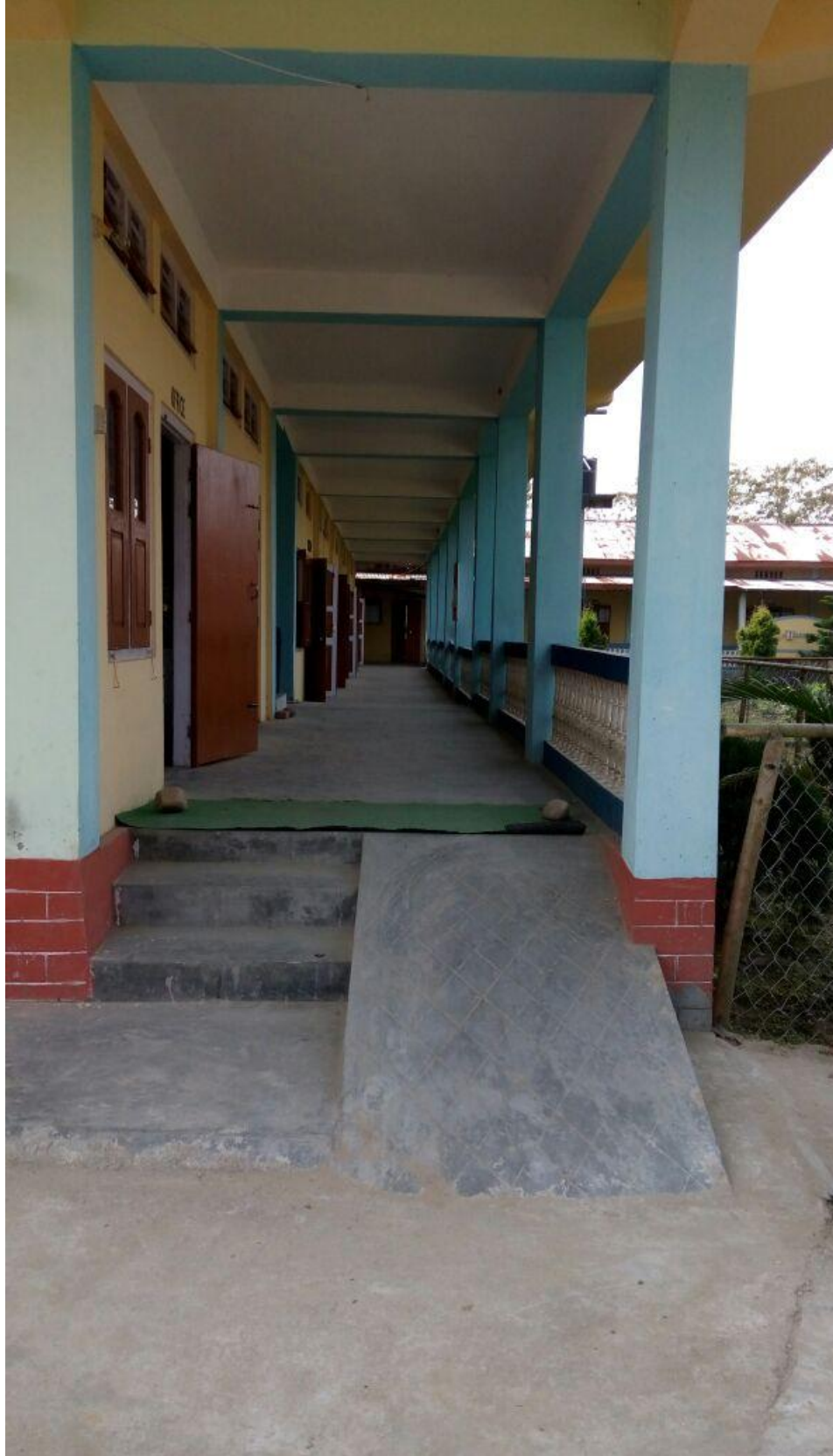
Staircase for Differently Abled Student at Departments' Common Room
