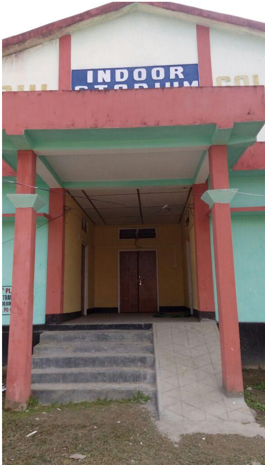
Staircase for Differently Abled Student at Indoor Stadium
