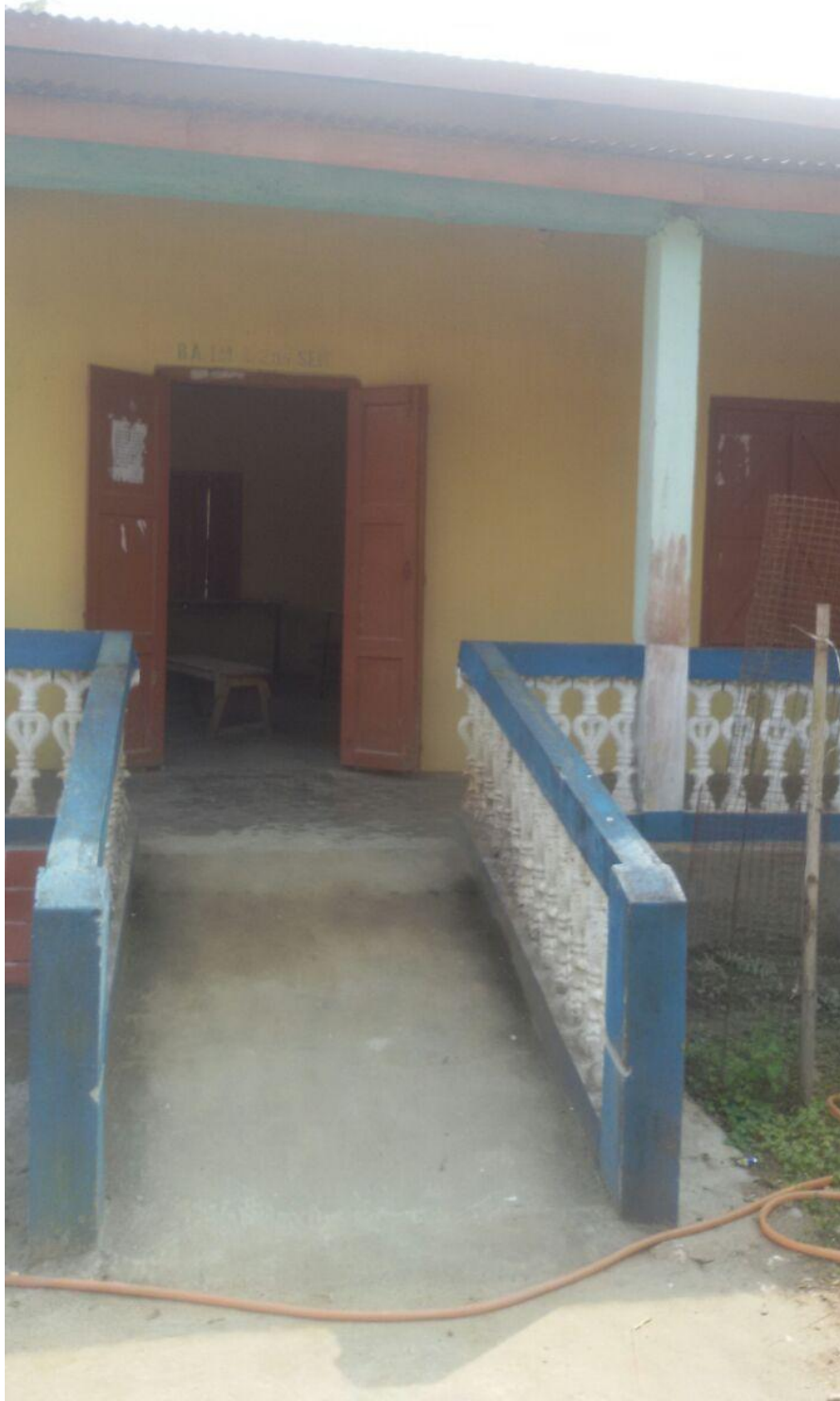
Staircase for Differently Abled Student in front of Classroom
